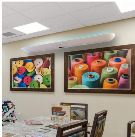
**265nm upper room ultraviolet germicidal irradiation (UVGI)** can disinfect the air in occupied spaces, autonomously and continuously reducing microbial counts in occupied spaces as individuals inhale and exhale air in shared spaces.\*
